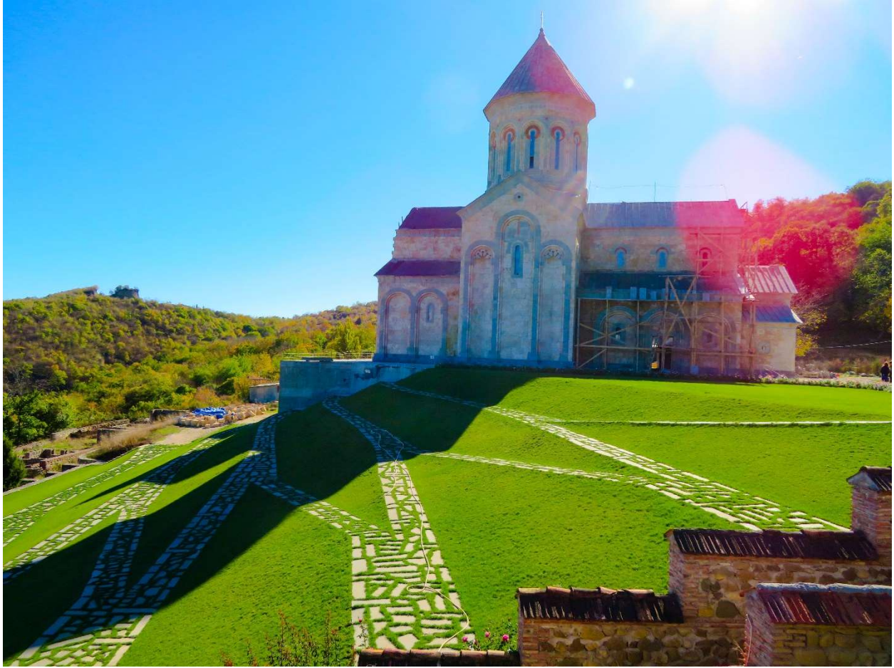
Signagi, A church is now under construction with a beautiful view
